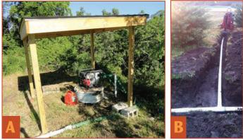
*Figure 8.* (A) A gas-powered 10 hp pump is covered to reduce wear from environmental damage and keep the engine cool during operation. (B) Belowground 3-inch PVC piping distributes water to various production fields.
