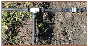
*Figure 6.* High pressure (50 psi) is maintained to distribute water with a pressure regulator (right) installed at the beginning of the header pipe. A garden hose thread connector at the end of the "T" allows for watering and overhead irrigation.
