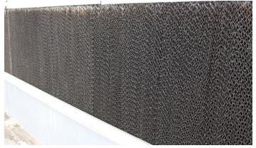
Figure 9. Algae accumulation on cellulose pads. (Photo: Raymond Cloyd)
