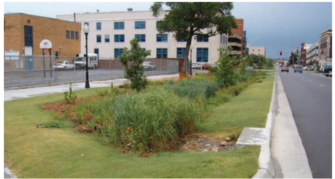
Figure 2. Native grass bioswale on Jackson Street near the state capitol building in Topeka.
